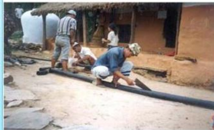
Constructing Modern RWH System in Nepal
