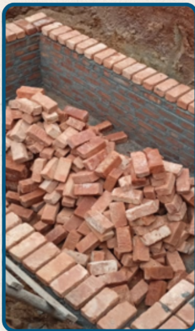
Underground sump being constructed
